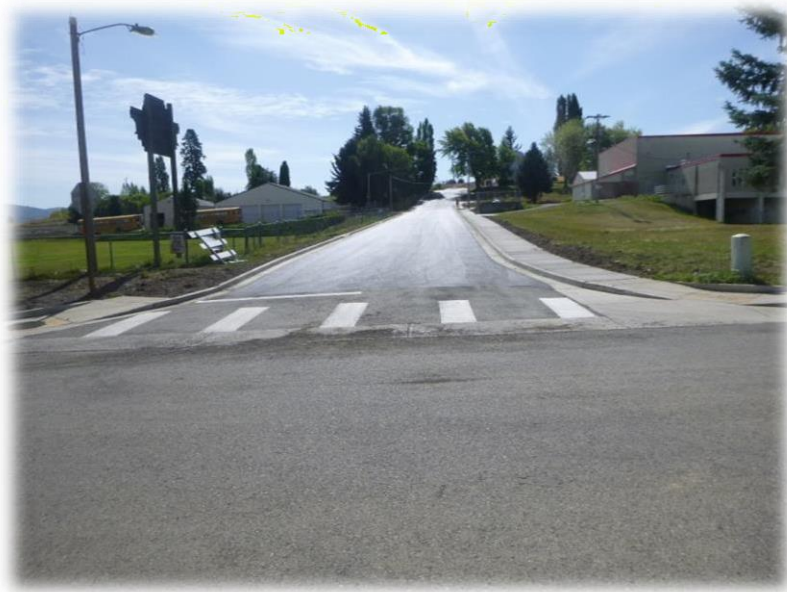
Davenport Way Road Completed in Summer 2019
