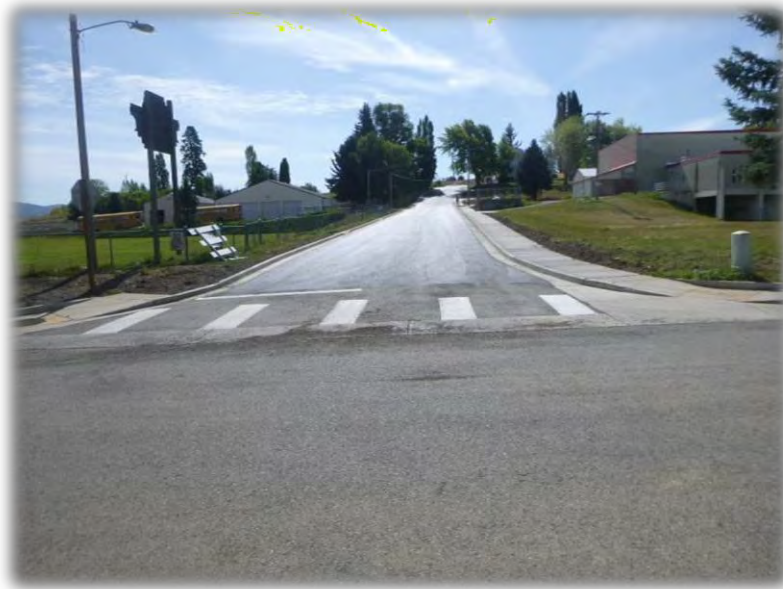
Davenport Way Road Completed in Summer 2019
