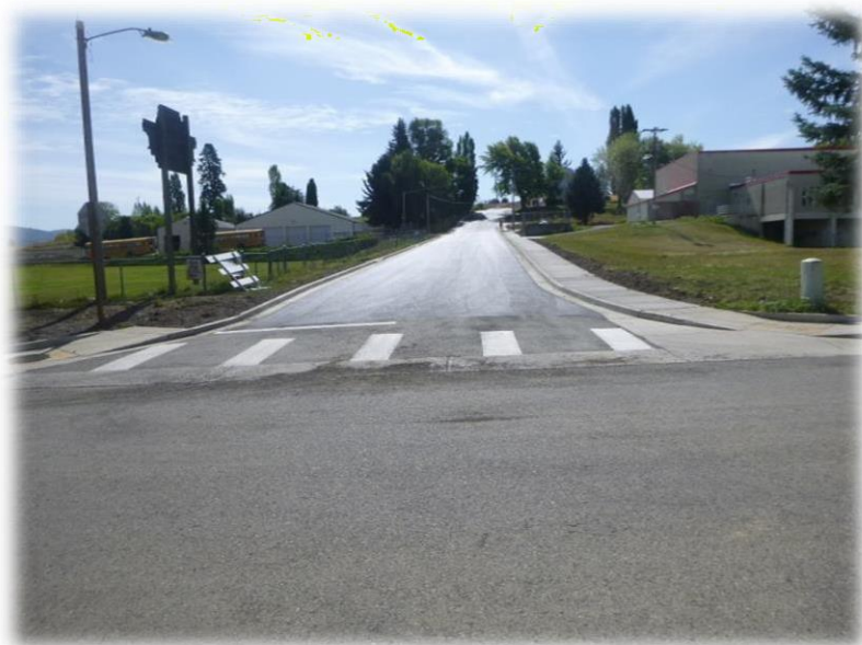
Davenport Way Road Completed in Summer 2019
