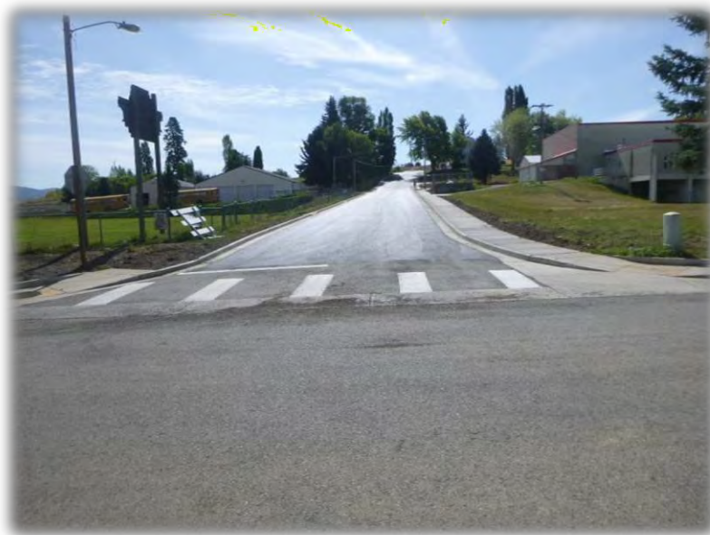
Davenport Way Road Completed in Summer 2019
