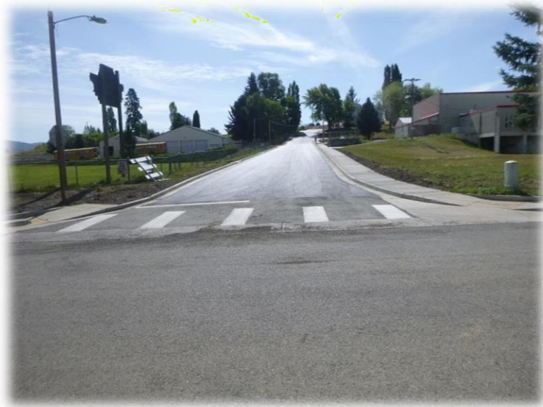
Davenport Way Road Completed in Summer 2019
