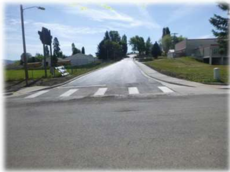
Davenport Way Road Completed in Summer 2019
