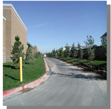
Secondary Access Road
