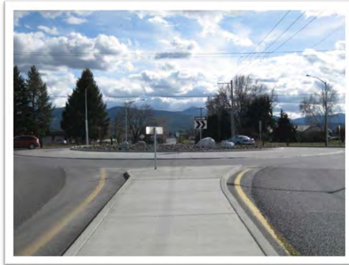
Prairie Ave. & McGuire Rd. Roundabout
