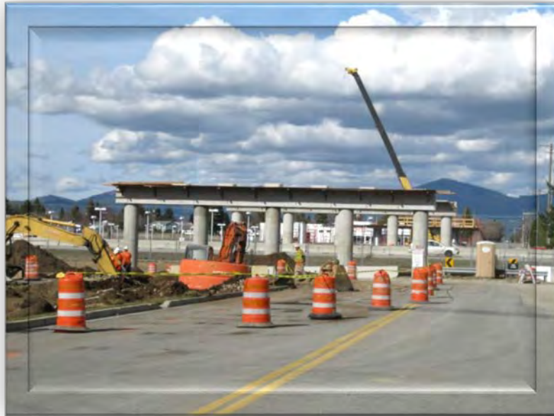
Greensferry Rd. Overpass Completed in 2015
